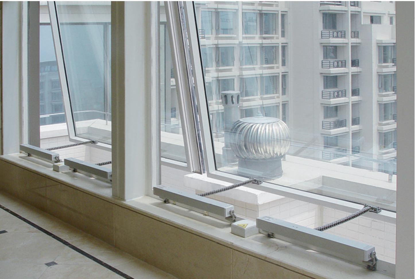
With a programme of different fanlight opening systems as well as chain and spindle drives, the Gretsche-Unitas group offers individual solutions for convenient daily ventilation.
