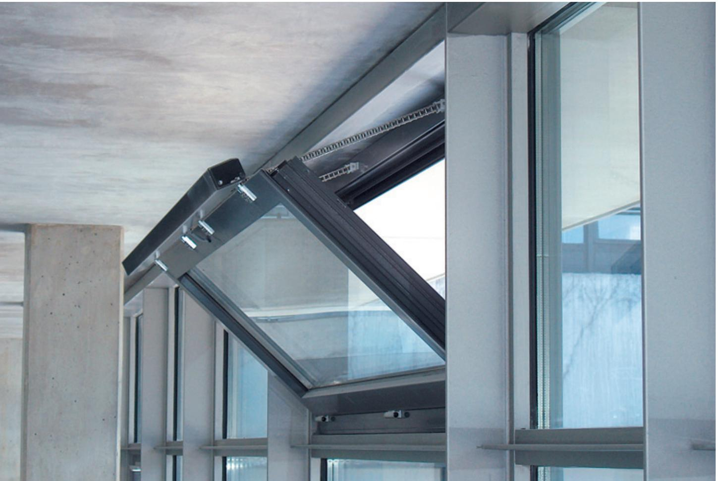
With their compact design and pleasant appearance, chain drives from the Gretsch-Unitas group are an ideal solution for the fast, electromotor-driven opening of exhaust air apertures and for room ventilation.
