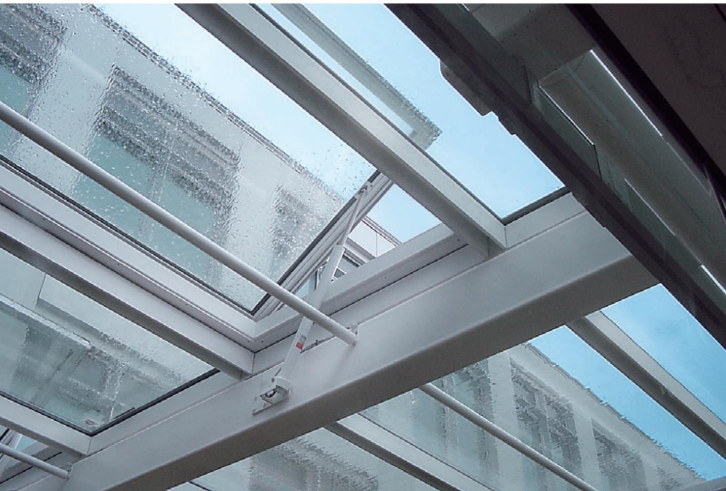
The spindle drives from the Gretsch-Unitas group are perfectly suited to opening and closing large and heavy skylights or facade openings.
