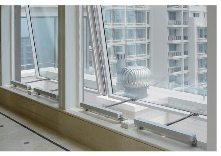
With a programme of different fanlight opening systems as well as chain and spindle drives, the Gretsch-Unitas group offers individual solutions for convenient daily ventilation.
