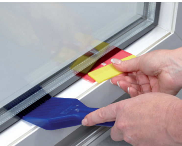
Glazing process – Insertion of the block
