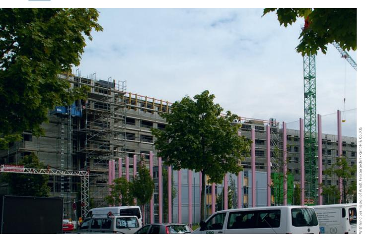
The energy balance of properties improves significantly when they are covered in a warm insulating layer. However, insulation not only changes the heat balance of a building, but also its structure: suddenly, the installation levels of windows and balcony-doors are no longer in masonry, but in the area of the insulation material. This cannot carry and transfer the loads.
