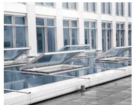
Heavyweight champion: ELTRAL S 80 can lift even large roof surface elements effortlessly
