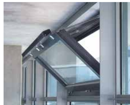
Chain drives with an integrated radio receiver can be activated individually or in groups via remote control
