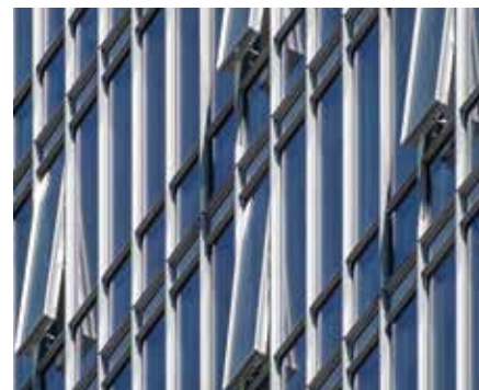
Sash heights of up to 2,500 mm are possible with bottom-hung windows
