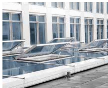
Skylight opening with spindle drive
