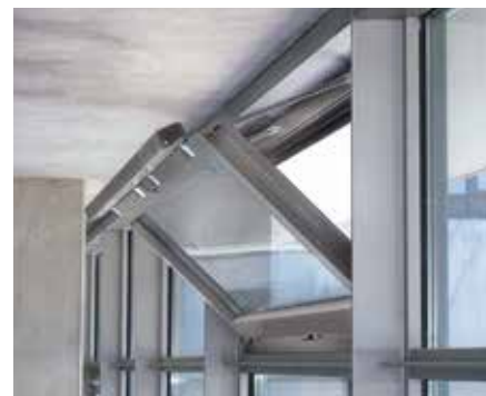
ELTRAL K60 Synchro: inward opening Tilt-Only sash, installation on sash
