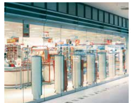
Multitude of individual partition walls and shop fronts for shop-in-shop concepts
